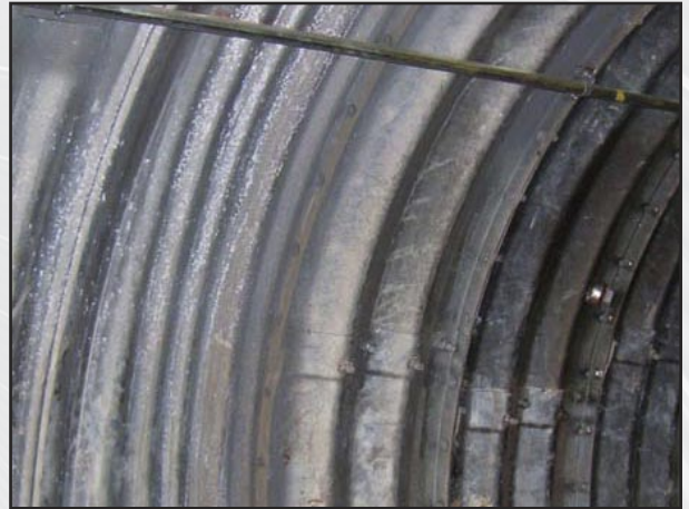
TUNNEL LINER PLATE WELDED TO CSP
