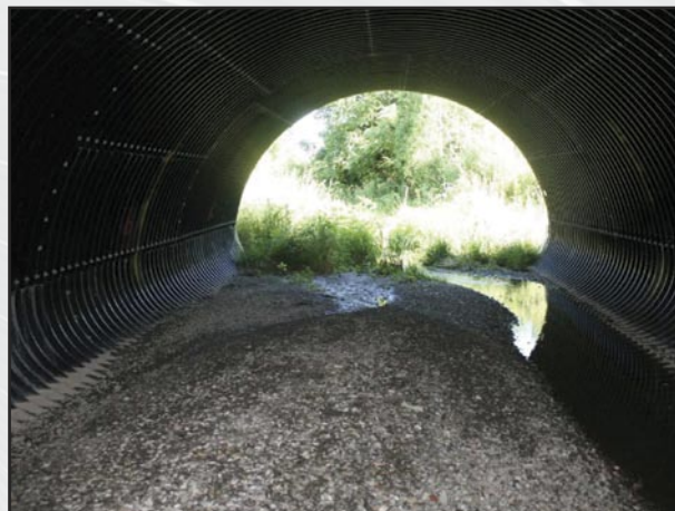
NATURAL GRAVEL IN-FILL OF POLYMER COATED STRUCTURAL PLATE PIPE-ARCH
