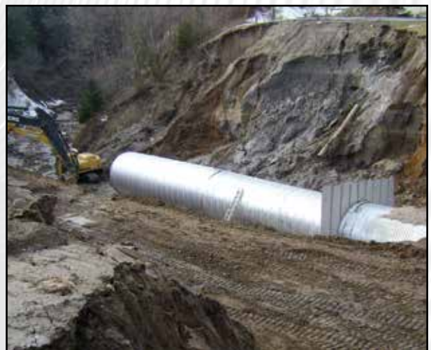
ANTI SEEP DIAPHRAGM ON DEEP FILL CULVERT
