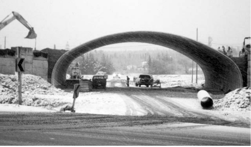
Long span structure under construction for grade separation.
