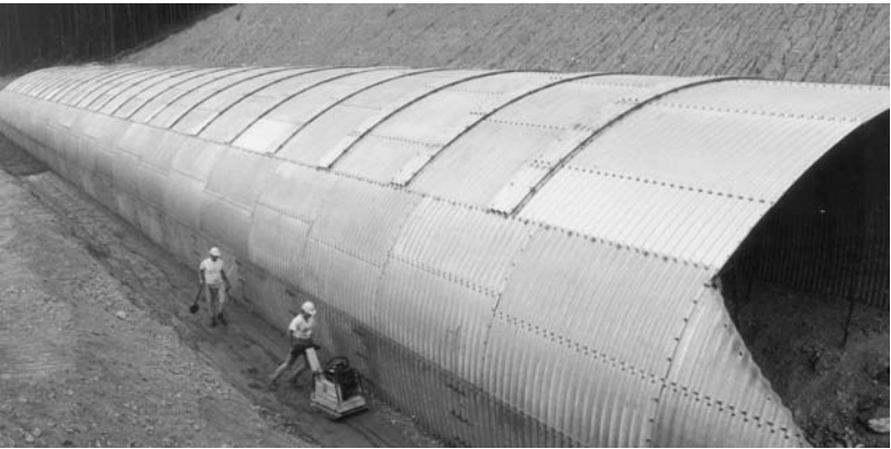
Backfilling adjacent to long-span structure with structural plate ribs.
