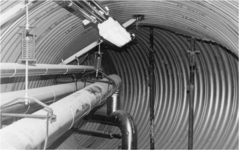
Corrugated pipe provides excellent conduit for utility lines.
