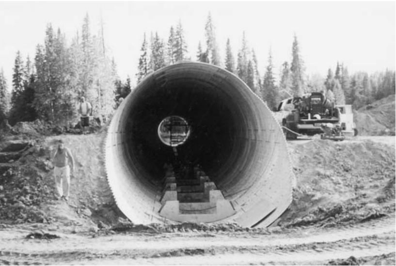
Structural plate pipe installation with fish baffles attached to invert.
