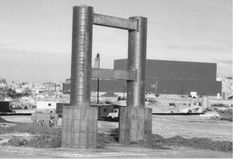
Ventilation ducts.
