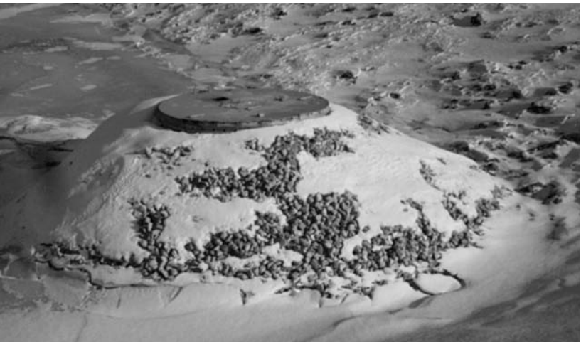
Perforated CSP riser surrounded by clear stone for storm water quality treatment and discharge quality control.
