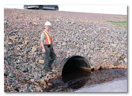
An engineer from a Member Company of the Corrugated Steel Pipe Institute inspects the new PLCSP culvert installation.
