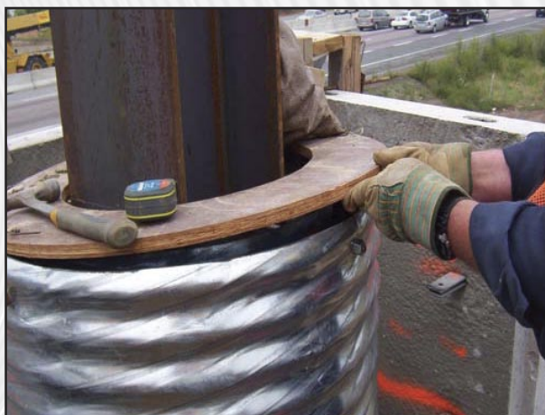
CLOSING IN THE CAISSON
