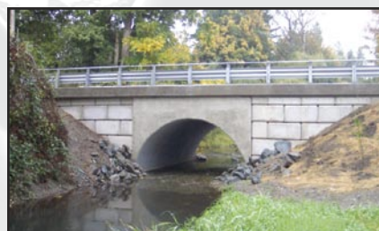
PIPE-ARCH CULVERT WITH BURIED INVERT ON WATERCOURSE
