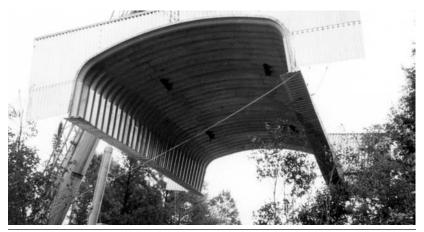
Lifting box culvert into place.
