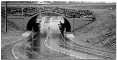
Long span structure for grade separation.
