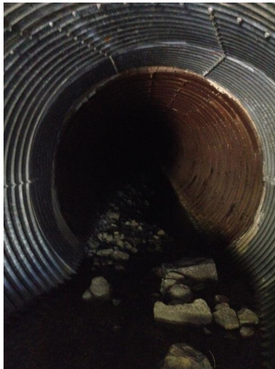
Figure 3.2 Transition from CSP to Liner Plate – July 2012
