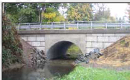
PIPE-ARCH CULVERT WITH BURIED INVERT ON WATERCOURSE
