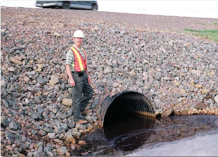
*An engineer from a Member Company of the Corrugated Steel Pipe Institute inspects the new PLCSP culvert installation.*
