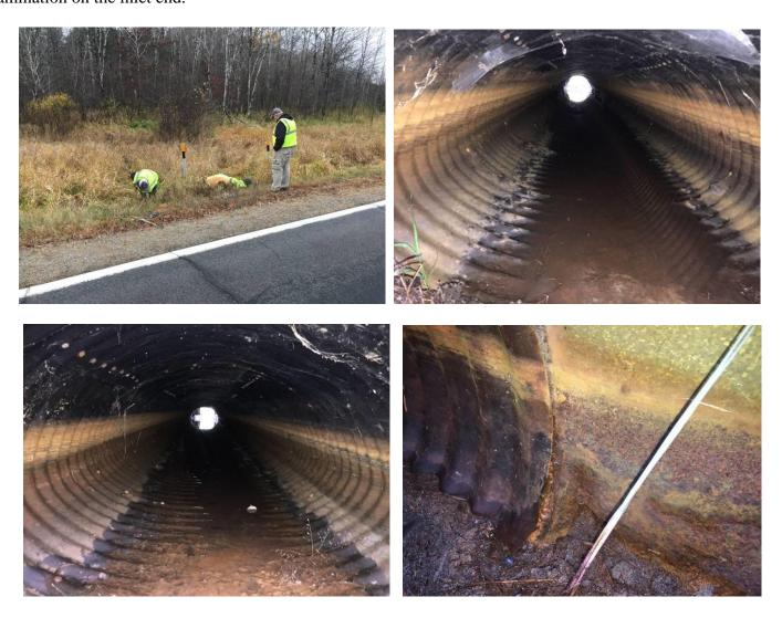
**Location #4** at mile post 2.73 – 42" X 29" Pipe Arch Shape Pipe Rating – Still Okay 2 (Fair - some wear, but structurally sound). The pipe appeared to be in good shape with minor delamination at a few riveted seams. The galvanized end section was rusted through.
