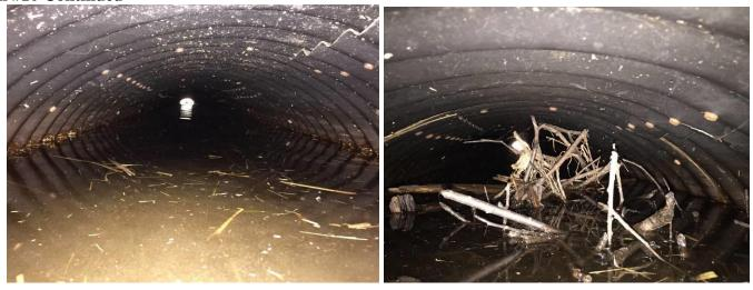
**Location #11** at mile post 21.84 – 28" X 20" Pipe Arch Shape Pipe Rating – Still Okay 2 (Fair - some wear, but structurally sound). There was sediment in the outlet end. Most of the pipe was free of sediment. The polymer coating was in good shape.
