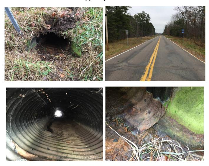
**Location #10** at mile post 19.27 – 28" X 20" Pipe Arch Shape Pipe Rating – Still Okay 2 (Fair - some wear, but structurally sound). Partially submerged with beaver dam on the outlet end. The polymer coating appeared to be in good shape in the invert when reaching through the water.
