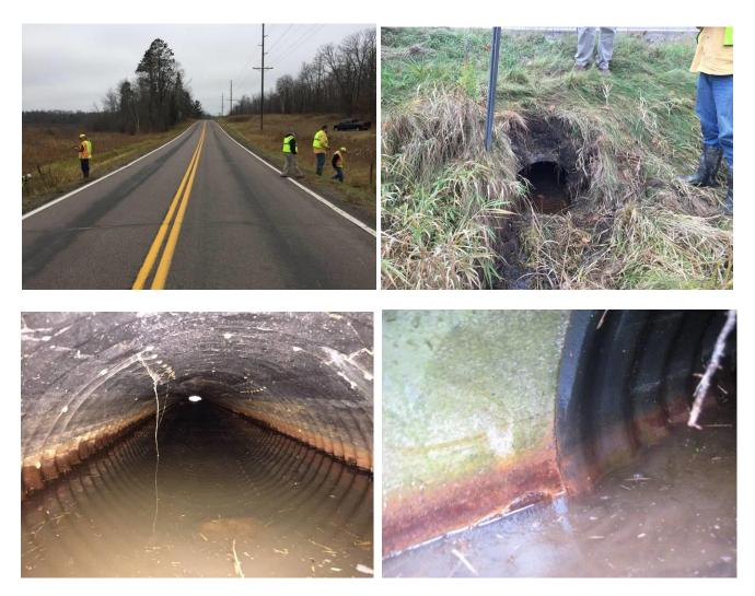
**Location #7** at mile post 18.48 - 28" X 20" Pipe Arch Shape Pipe Rating – Still Okay 2 (Fair - some wear, but structurally sound). The pipe was in good shape with minor delamination on the inlet end and at a few seams. The galvanized end section was rusty through.
