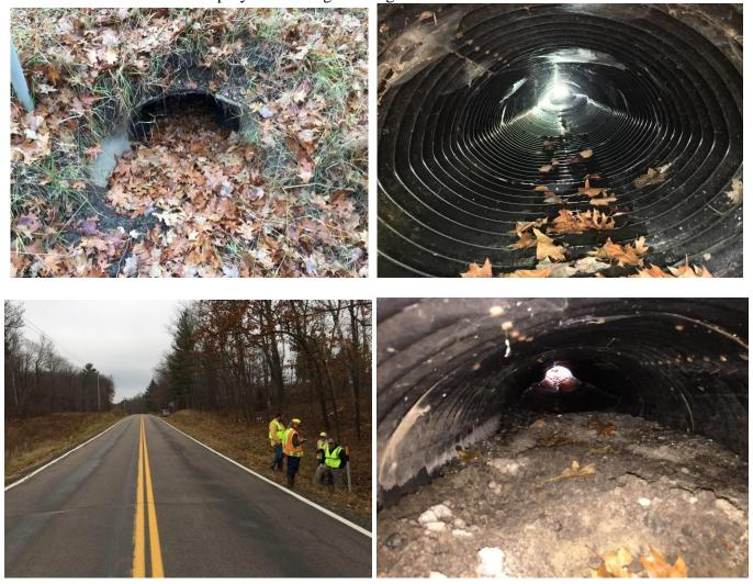
**Location #13** at mile post 29.13 – 28" X 20" Pipe Arch Shape Pipe Rating – Still Okay 2 (Fair - some wear, but structurally sound). Dry with moist sediment on outlet end. The polymer coating was in good condition. The end section shows corrosion with high water line.
