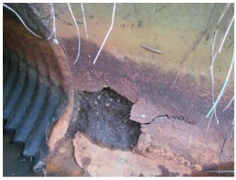
**Location #5** at mile post 12.81 - 28" X 20" Pipe Arch Shape Pipe Rating – Still Okay 2 (Fair - some wear, but structurally sound). There was delamination throughout the culvert, however no perforations were in the base steel of the culvert. The galvanized end section did show corrosion with pitting through the steel.
