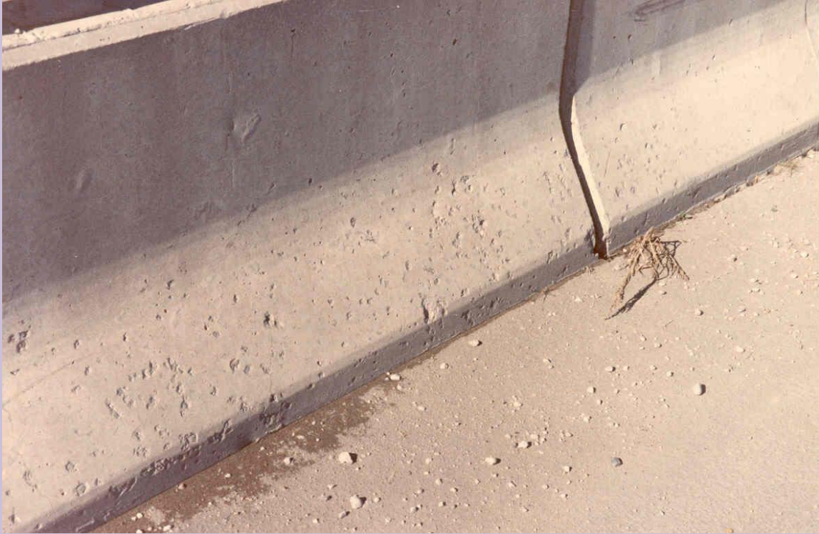
Figure 2. Example of Light Scaling
