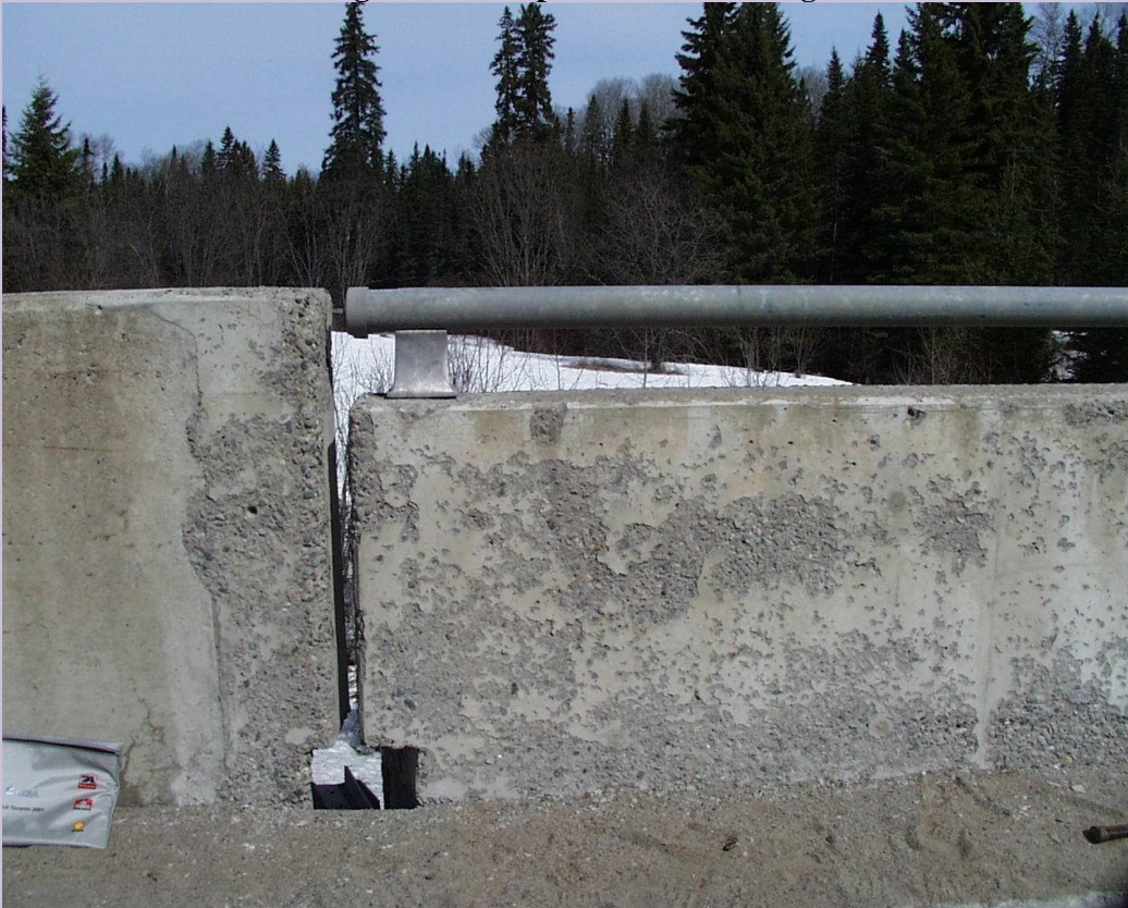
Figure 6. Example of Severe Scaling
