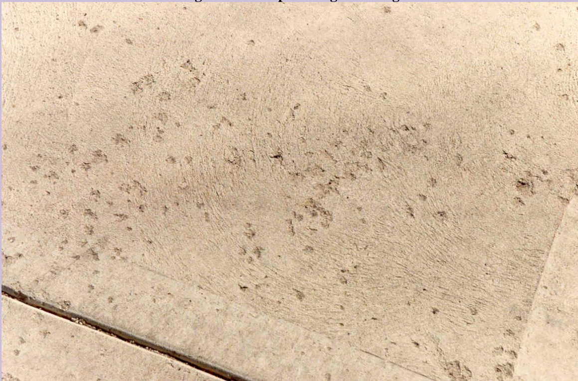
Figure 2. Example of Light Scaling
