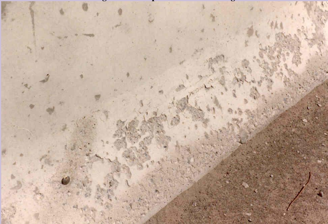
Figure 4. Example of Medium Scaling
