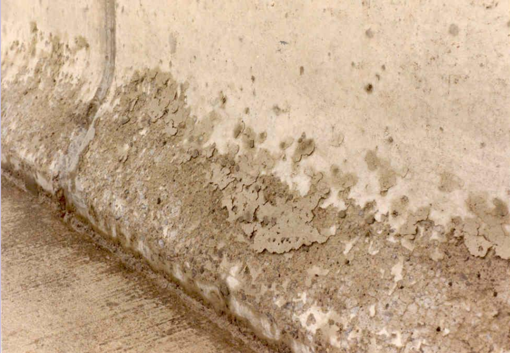
Figure 6. Example of Severe Scaling
