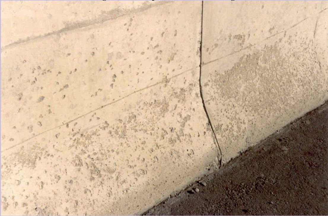
Figure 4. Example of Medium Scaling
