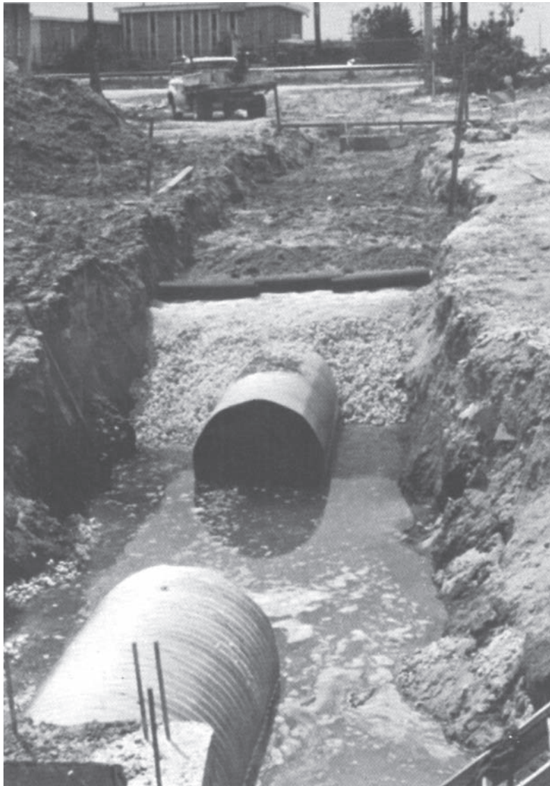
Common recharge trench installation showing relative placement of perforated pipe ballast rock, gravel, and asphalt impregnated building paper.
