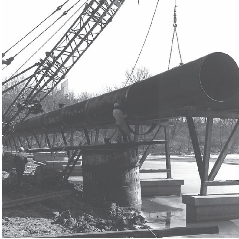
CSP aerial sewer being installed.
