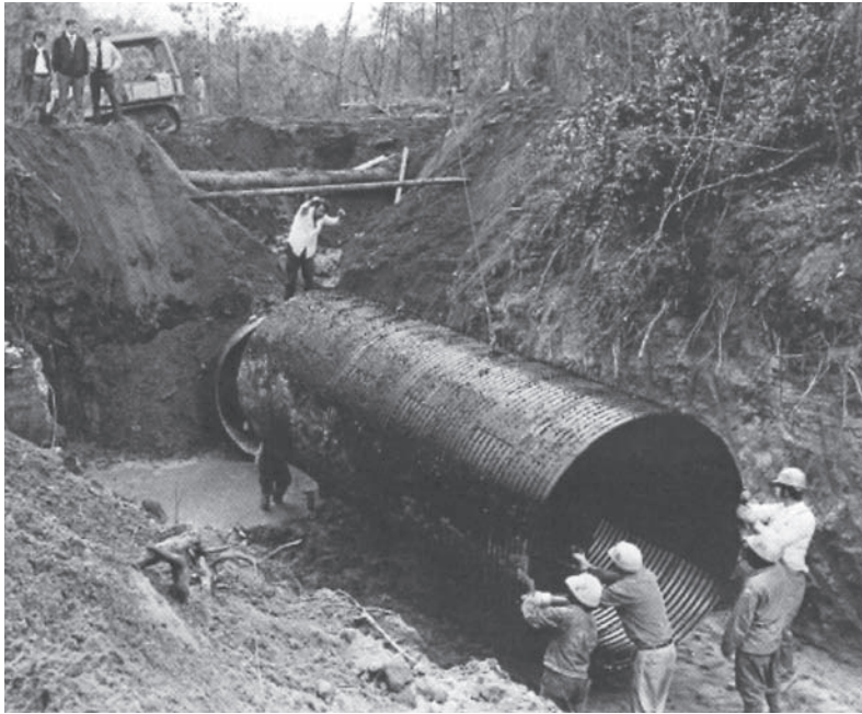
Speed and ease of installation is a major factor in the choice of CSP for storm drainage.
