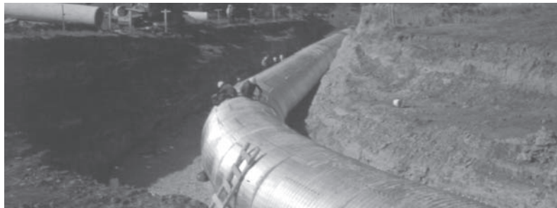
Installation of SPCSP.
