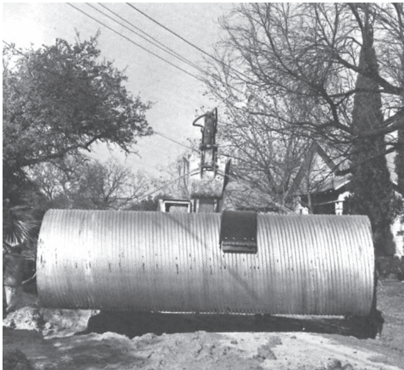
Installing a fully paved sanitary sewer.
