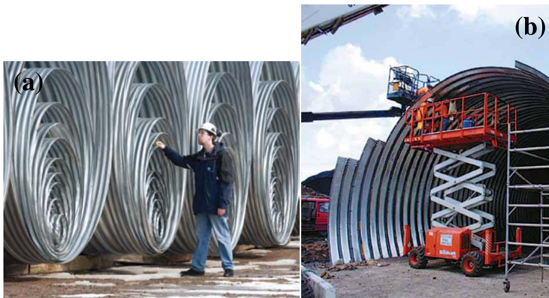
FIGURE 1 (a) Corrugated steel pipe. (b) Structural plate corrugated steel pipe (5).
