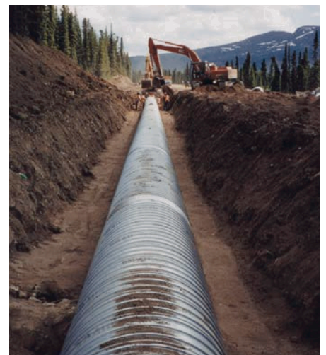
LONG LENGTHS AND POSITIVE JOINTS ASSURE GOOD ALIGNMENT AND LEAK RESISTANT PERFORMANCE
