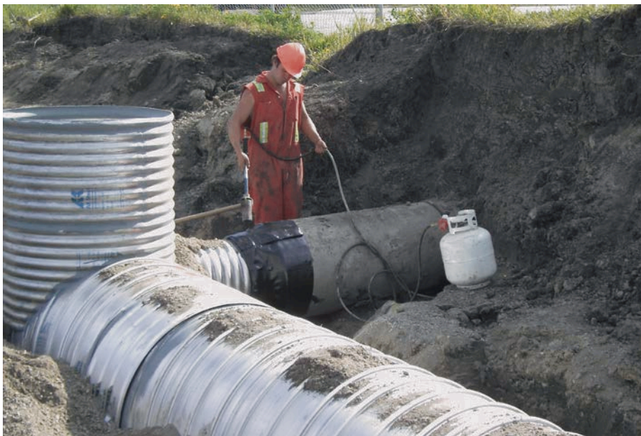
AN ULTRA FLO TEE-TYPE MANHOLE RISER COMBINED WITH A SERVICE TEE IS SHOWN COMBINING A STANDARD HEL-COR STUB WITH AN ULTRA FLO STORM SEWER PIPE
