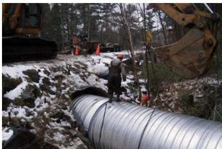
A HUGGER BAND COUPLER IS TIGHTENED AROUND PIPE ENDS TO PRODUCE A VERY STRONG JOINT
