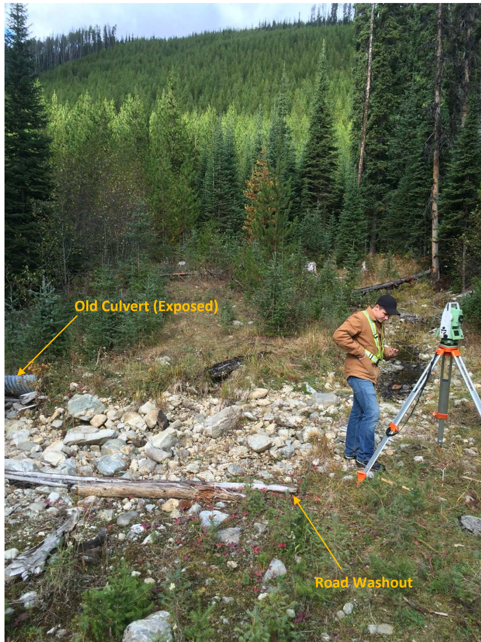
Fig. 2 – Derickson Rd. Washout at Tributary 3. (Taken by Eric)
