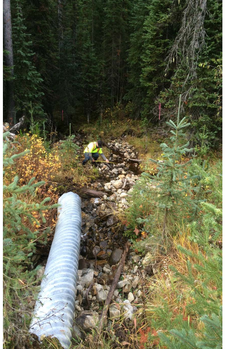
Fig. 4 – Downstream of Crossing/Culvert Washout (Taken by Eric)
