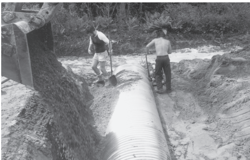
Backfill placement and compaction.
