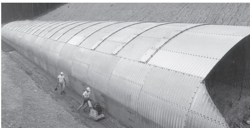
Backfilling adjacent to long-span structure with structural plate ribs.
