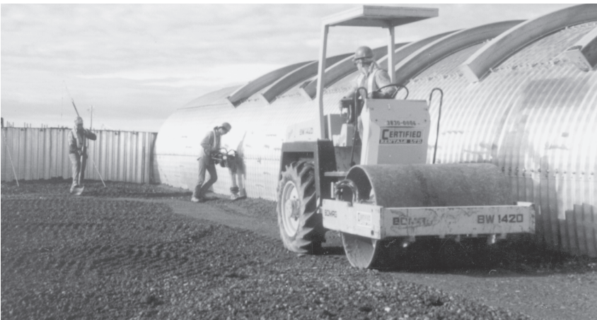
Backfill compaction adjacent to long span structural plate.
