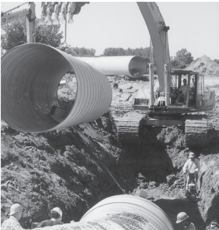
Lifting spiral rib pipe into place.
