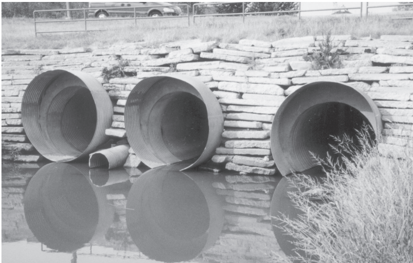
Improving hydraulic capacity (inlet control) with special features.
