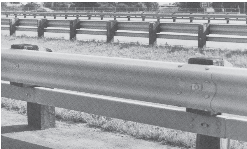
Offset mounting of W-beam on wood post.
