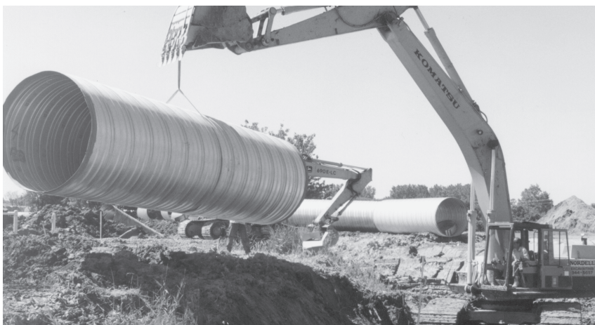
Lifting spiral rib pipe into place.
