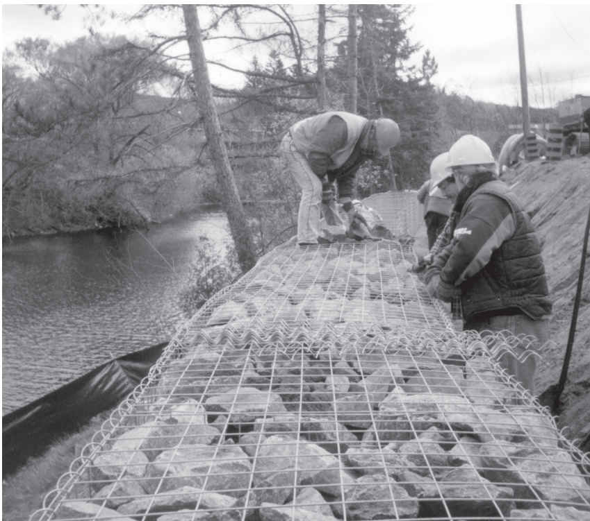
Construction of gabion wall.
