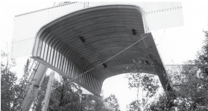
Lifting box culvert into place.
