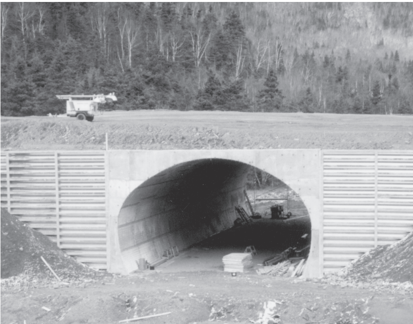
Long-span high profile arch with concrete and bin-type retaining wall headwall.
