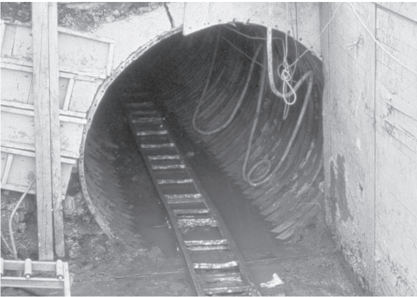
Liner plate tunnel entrance.
