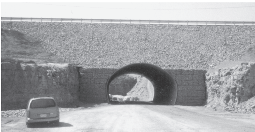
Quarry underpass under high cover.
