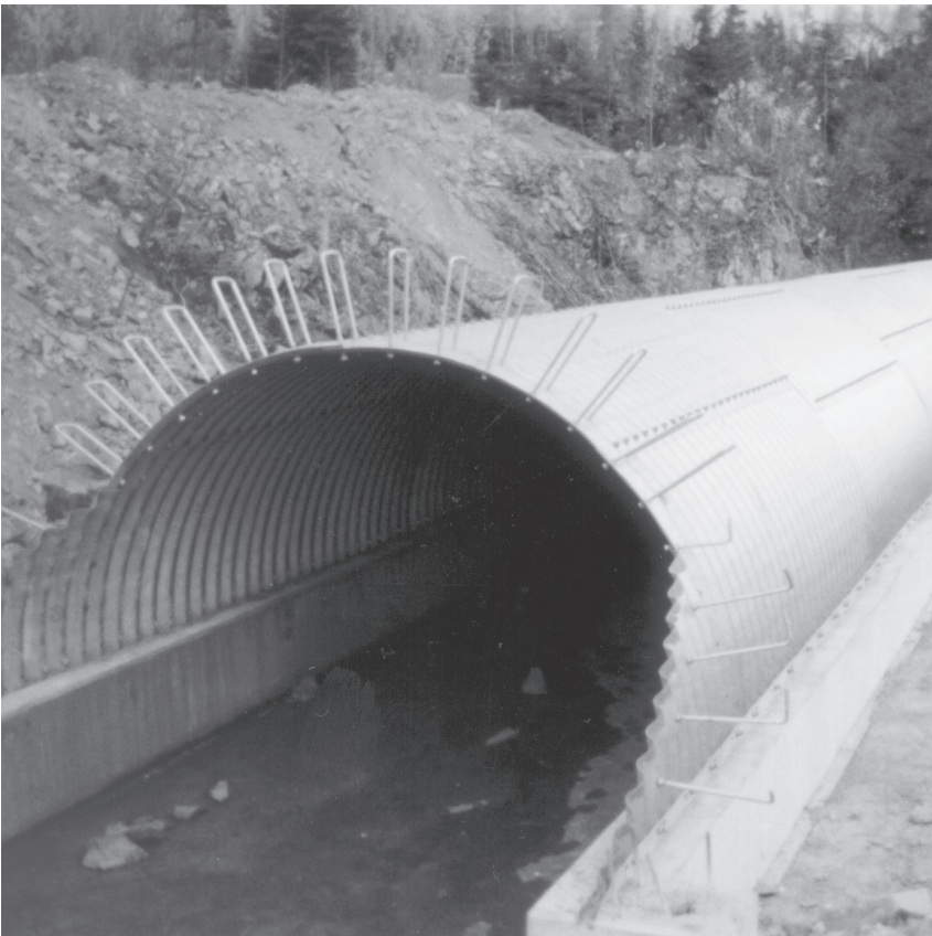
CSP structure ready for backfill placement and headwalls.
