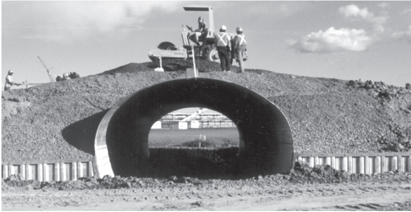
Compacting backfill over high-profile arch.
