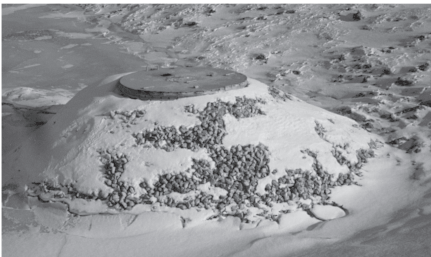
Perforated CSP riser surrounded by clear stone for storm water quality treatment and discharge quality control.
