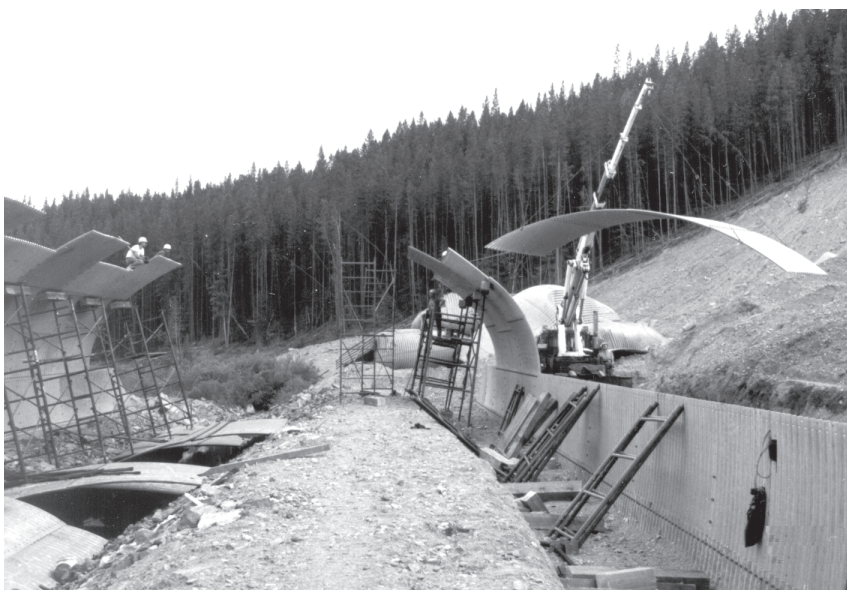
Lifting pre-assembled side plates into place.
