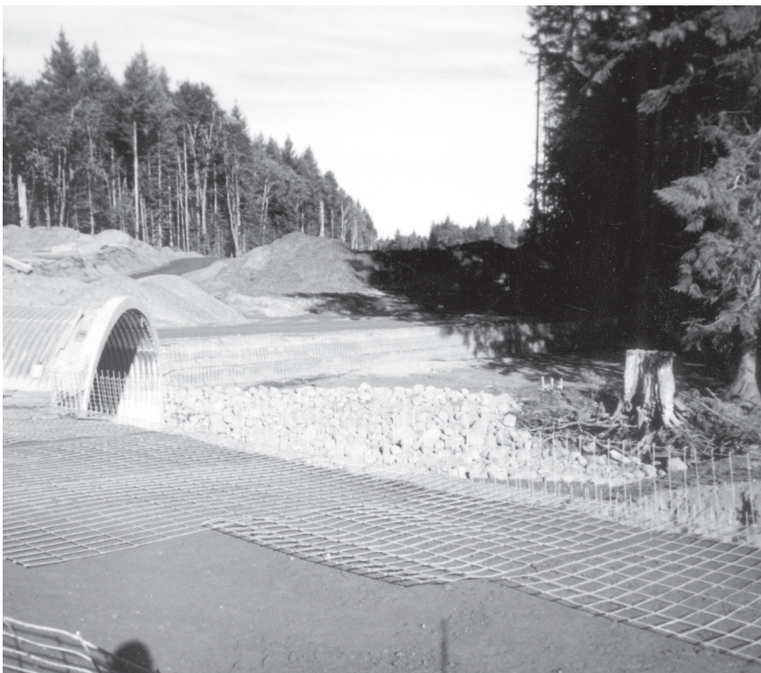
Construction of welded wire wall.
