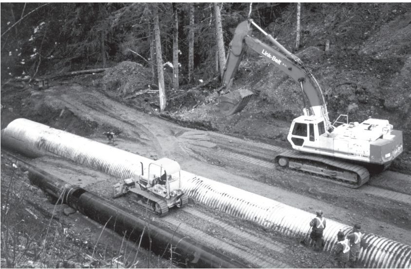
CSP installation with straight alignment.
