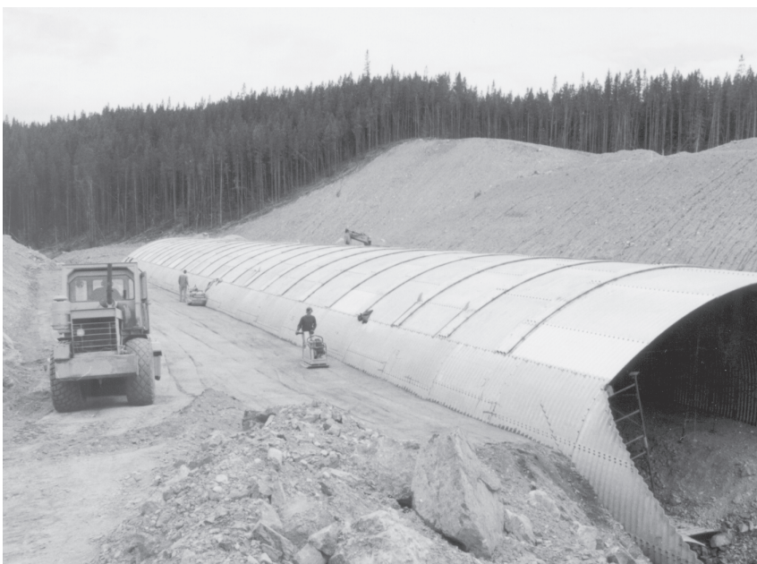
Backfill proceeds parallel to structure.
