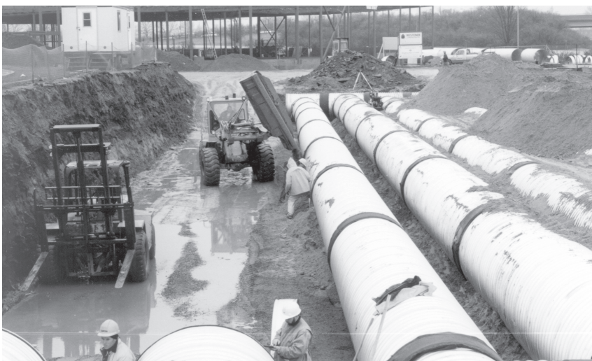
Backfilling stormwater detention system.
