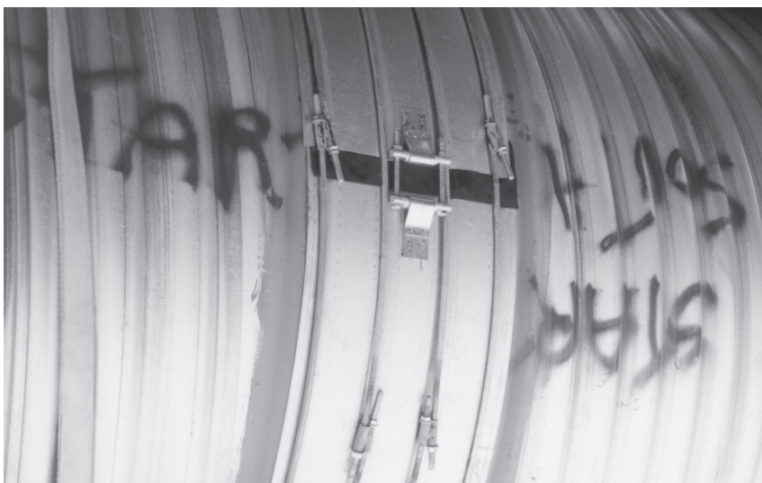
Combination dog bone, and rod and lug coupler.
