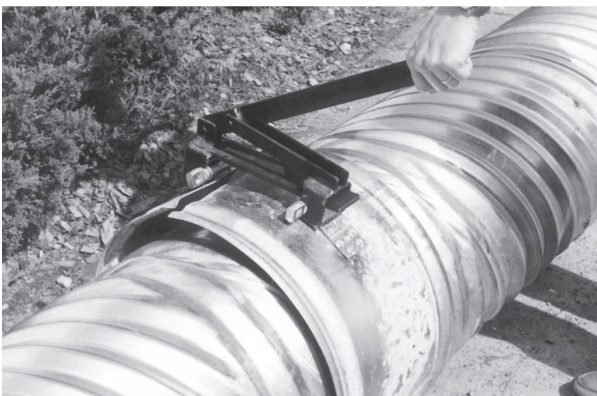
A band puller eases installation of coupler.
