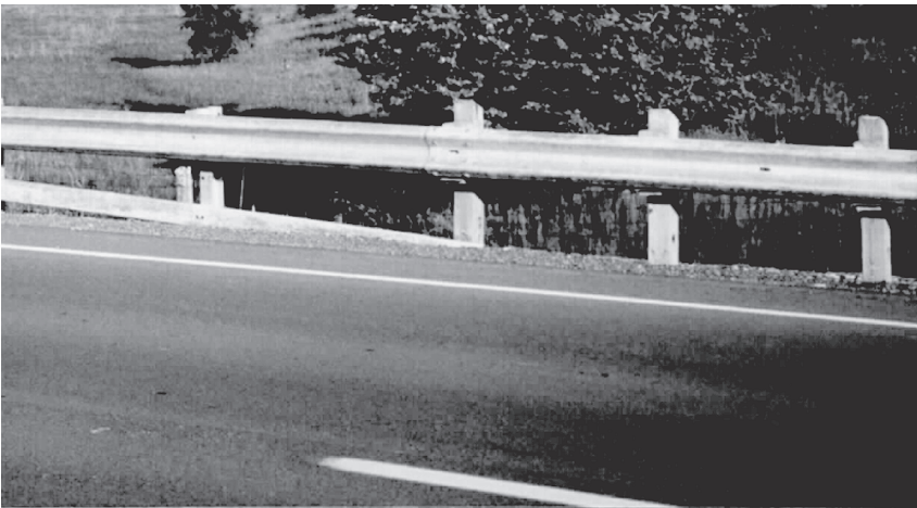
Transition of rub-rail channel with W-beam guiderail system.
