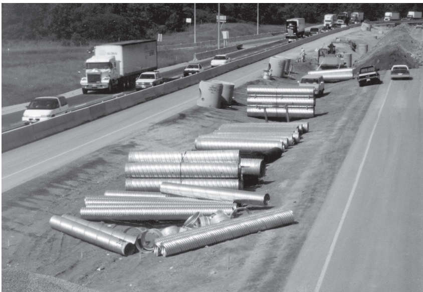
Highway 401 in Ontario using spiral rib steel pipe and corrugated steel pipe for median drainage.
