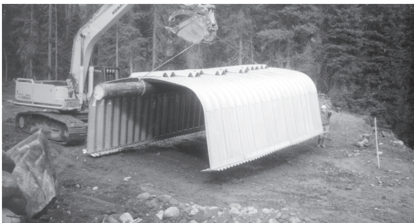
Deep corrugated structural plate box culvert assembled at job site.
