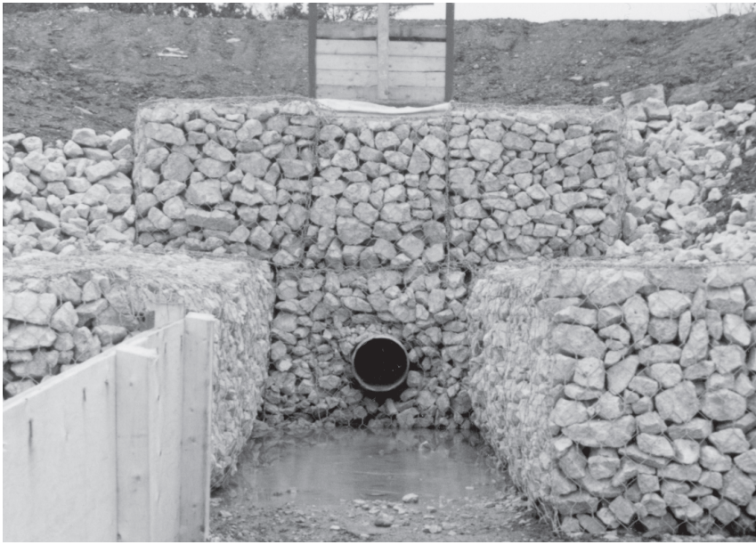
Gabions provide protection.
