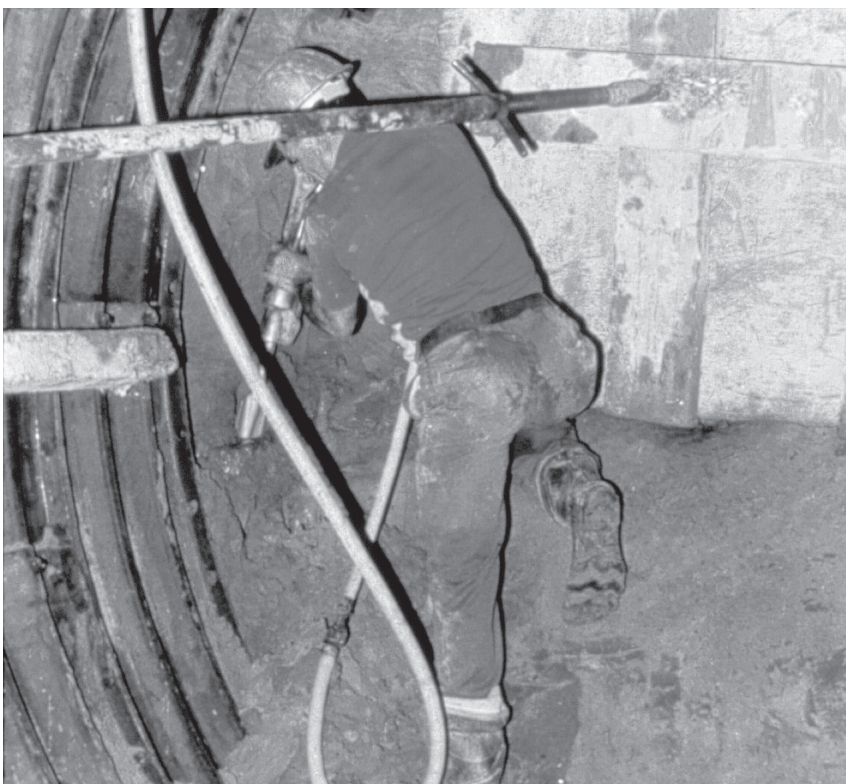
Liner plate shaft construction.
