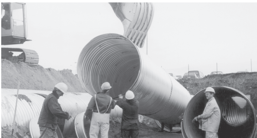
Lifting CSP into place.
