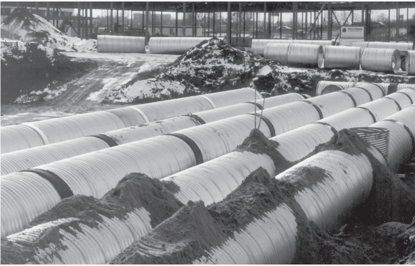
Stormwater detention system.
