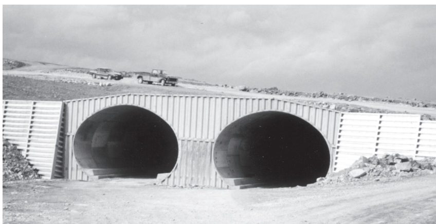
Twin high-profile arch mine underpass, with sheeting and bin-type retaining wall end treatment.
