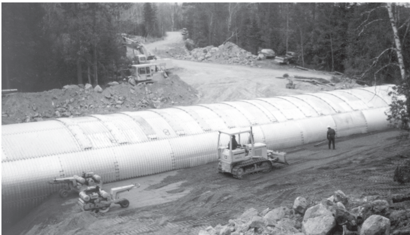
Backfilling long span structure with structural plate ribs.
