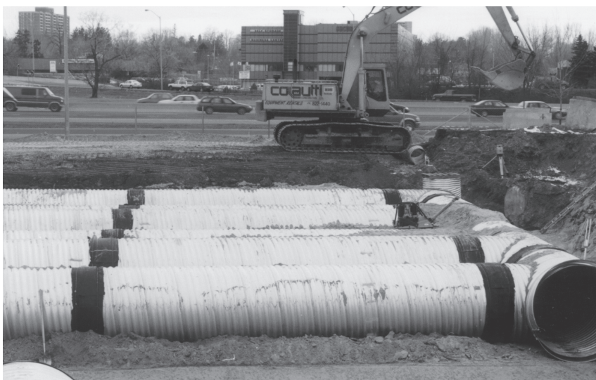
Joints wrapped with geotextile to prevent migration of fines into the pipes.
