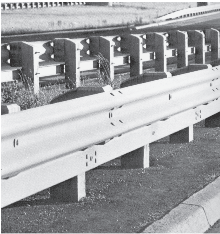
W-beam guiderail with channel rub rail located below.
