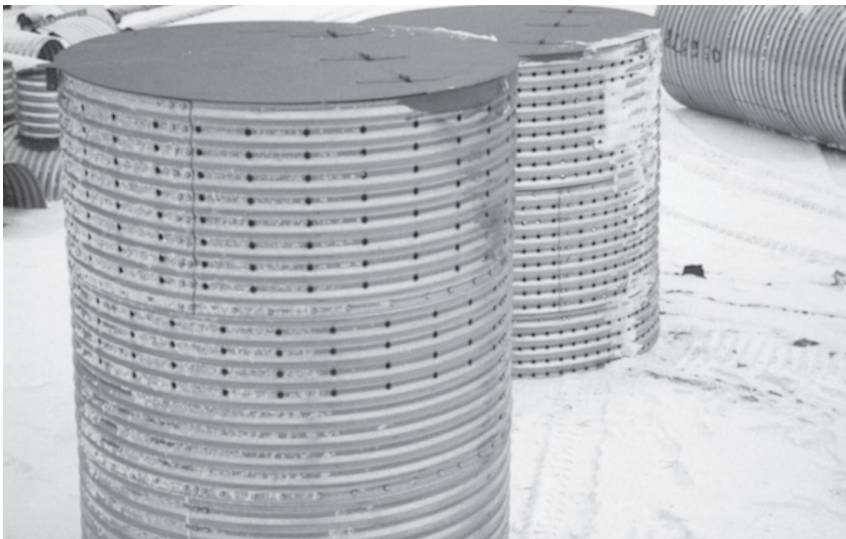
Perforated pipe for storm water management pond discharge treatment and quality control.
