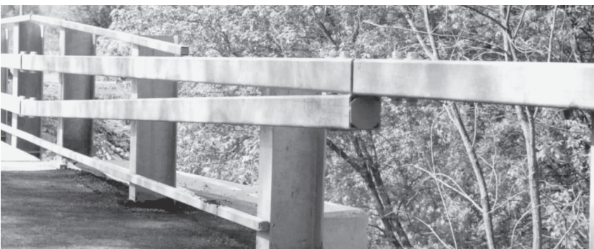
Transition from bridge rail to box-beam guiderail.
