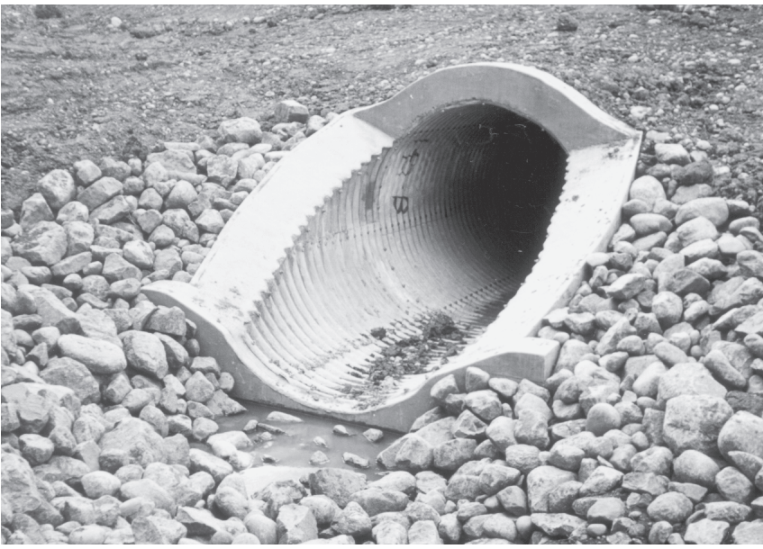
Structural plate CSP with concrete end treatment.
