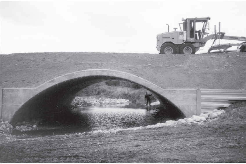
Low profile arch with concrete and bin-type retaining wall end treatment.
