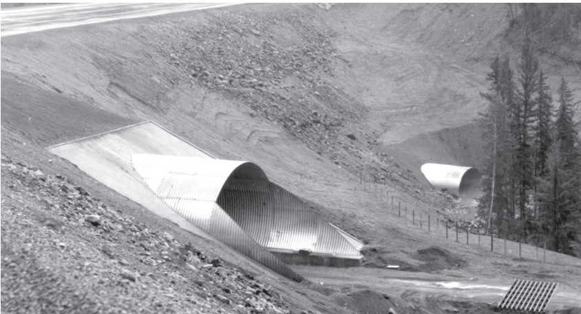
Structural plate underpass and stream crossing. The sizes of these structures are 11.69 m span x 7.42 m rise horizontal ellipse and 6.94 m diameter round pipe respectively. The round pipe had 28.2 m of cover.
