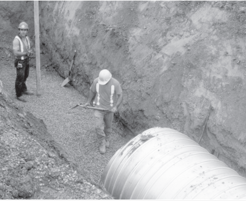
Placing and checking of elevation of pipe bedding.
