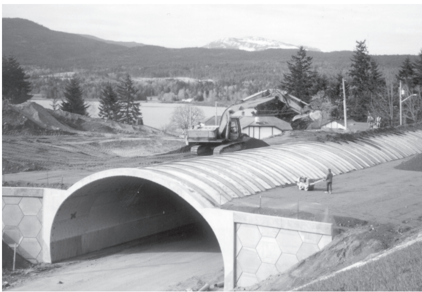
Backfilling high-profile highway underpass.
