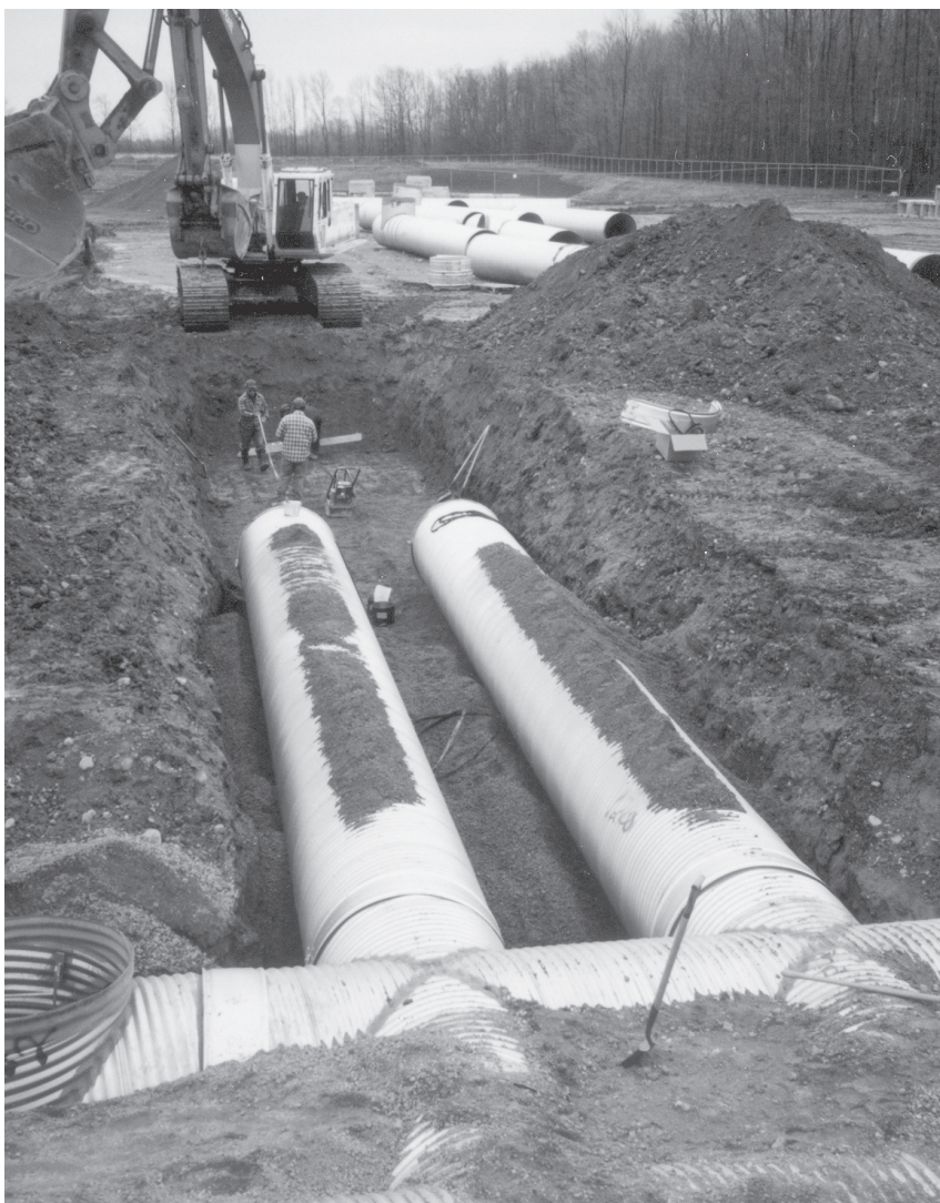
Stormwater detention system installation.
