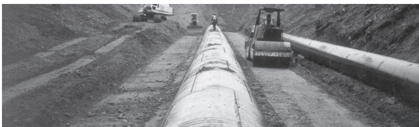
Compaction parallel to pipe.
