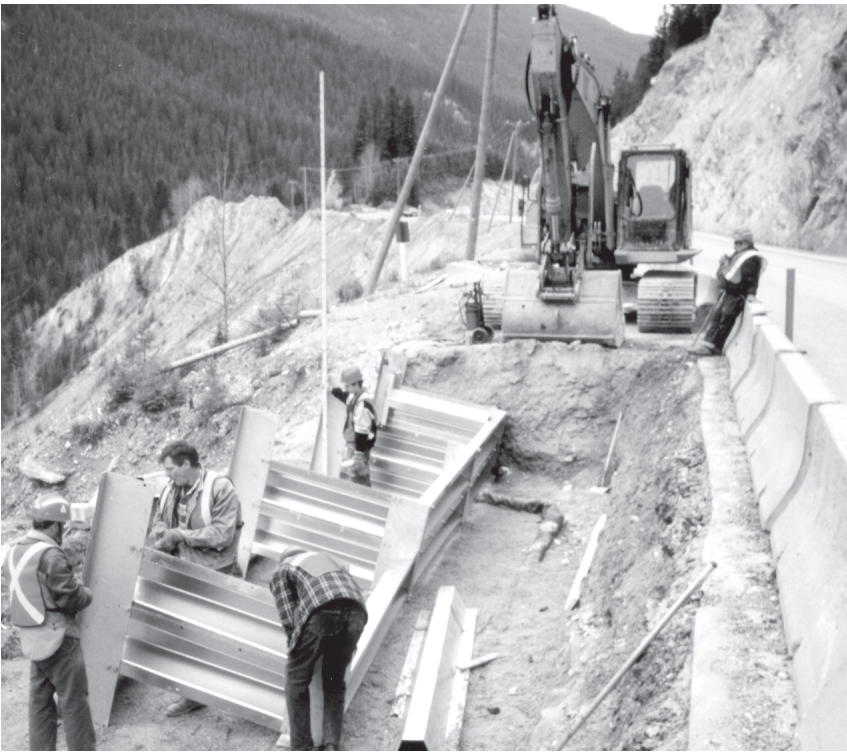
Bin type retaining wall being assembled.
