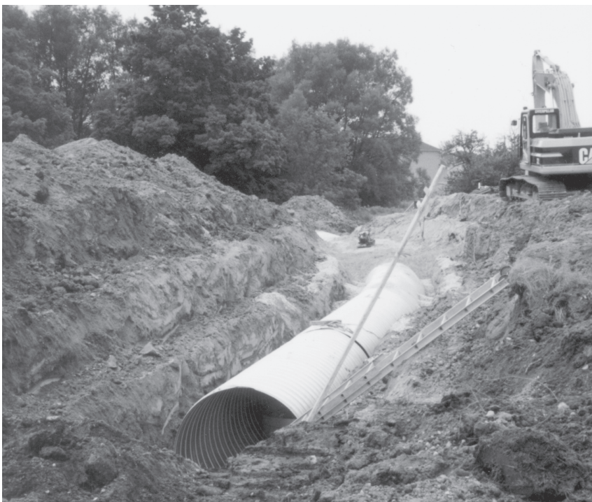
Spiral rib steel pipe stream diversion installation.
