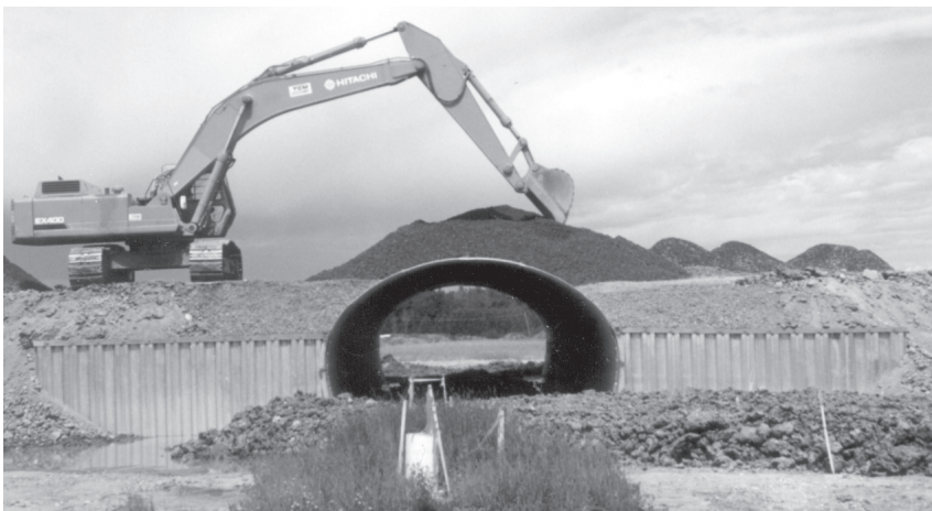
Cold-formed sheet steel piling prevents erosion.
