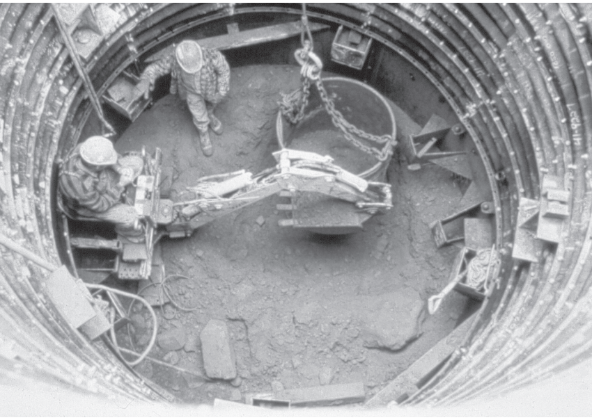
Liner plate shaft construction.
