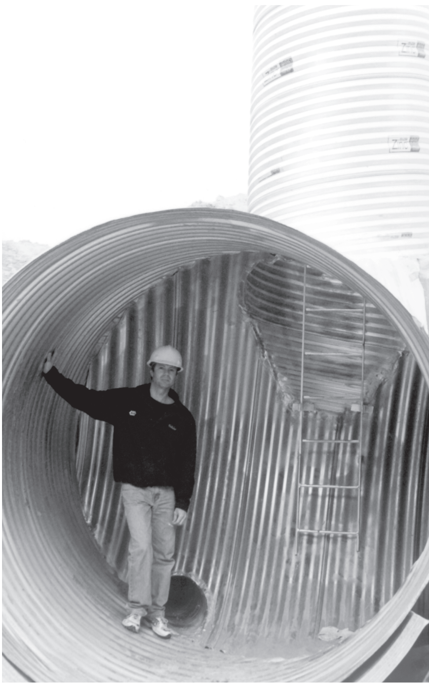
Fabricated riser type CSP manhole.
