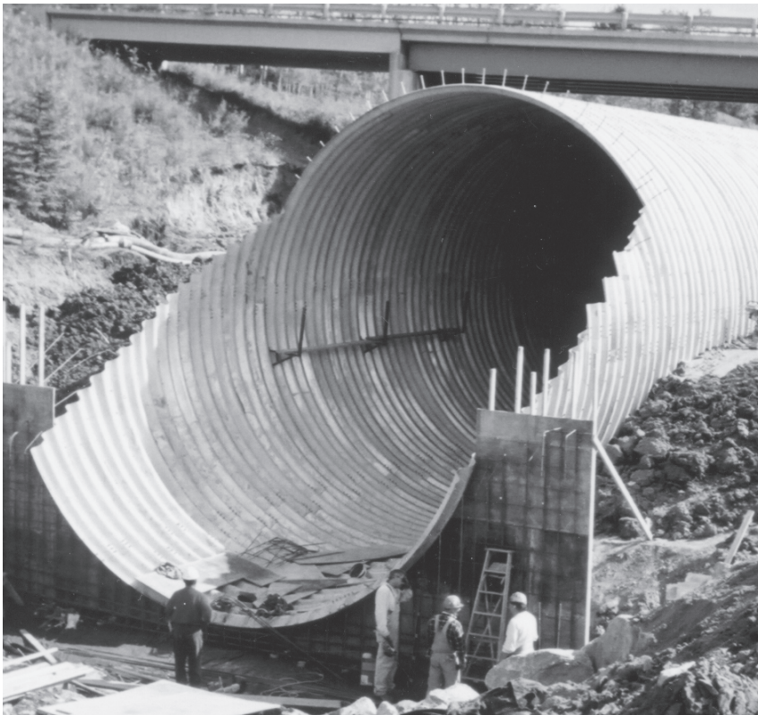
Installation of large diameter pipe with step-beveled end.
