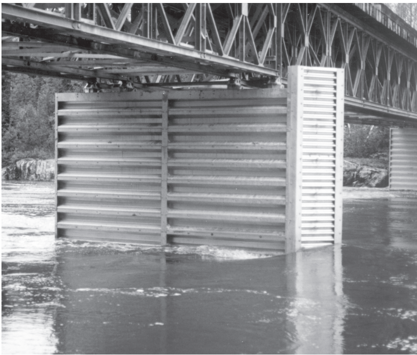
Bridge pier uses bin type retaining wall components.
