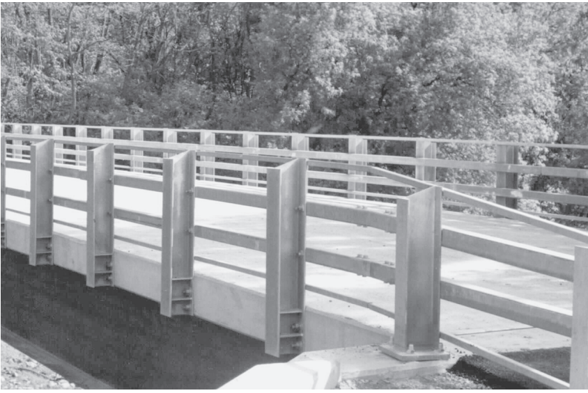
Typical bridge tubular steel railing.
