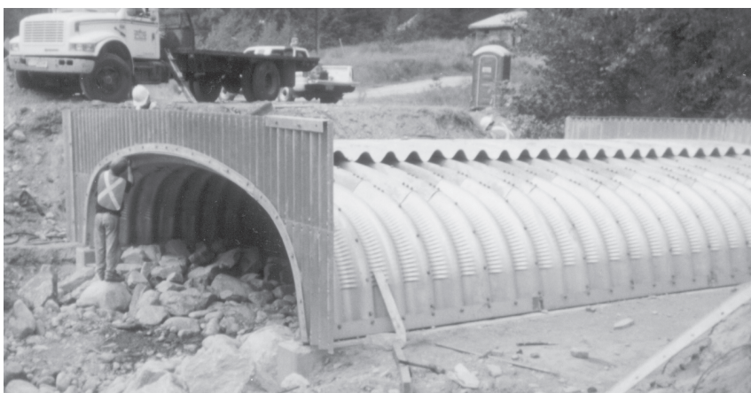
Deep corrugated structural plate box culvert on foundation with end walls attached.
