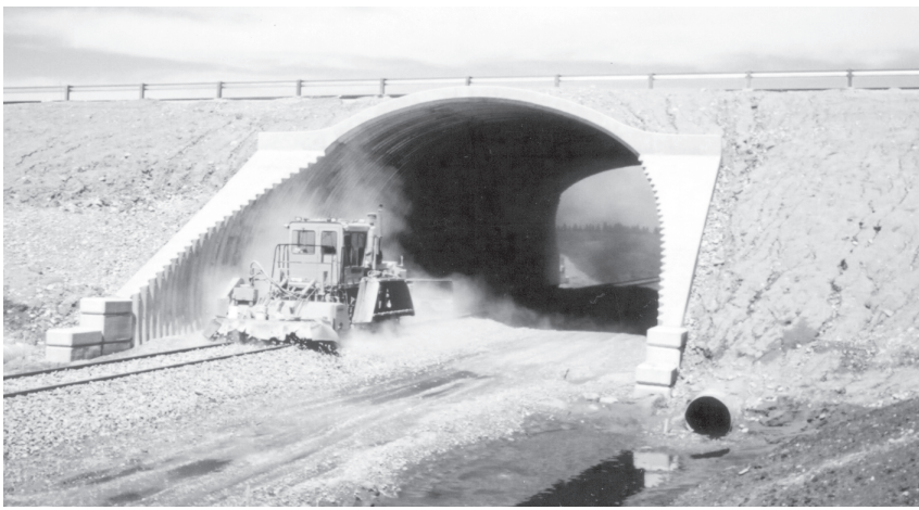
End treatment of large structure.
