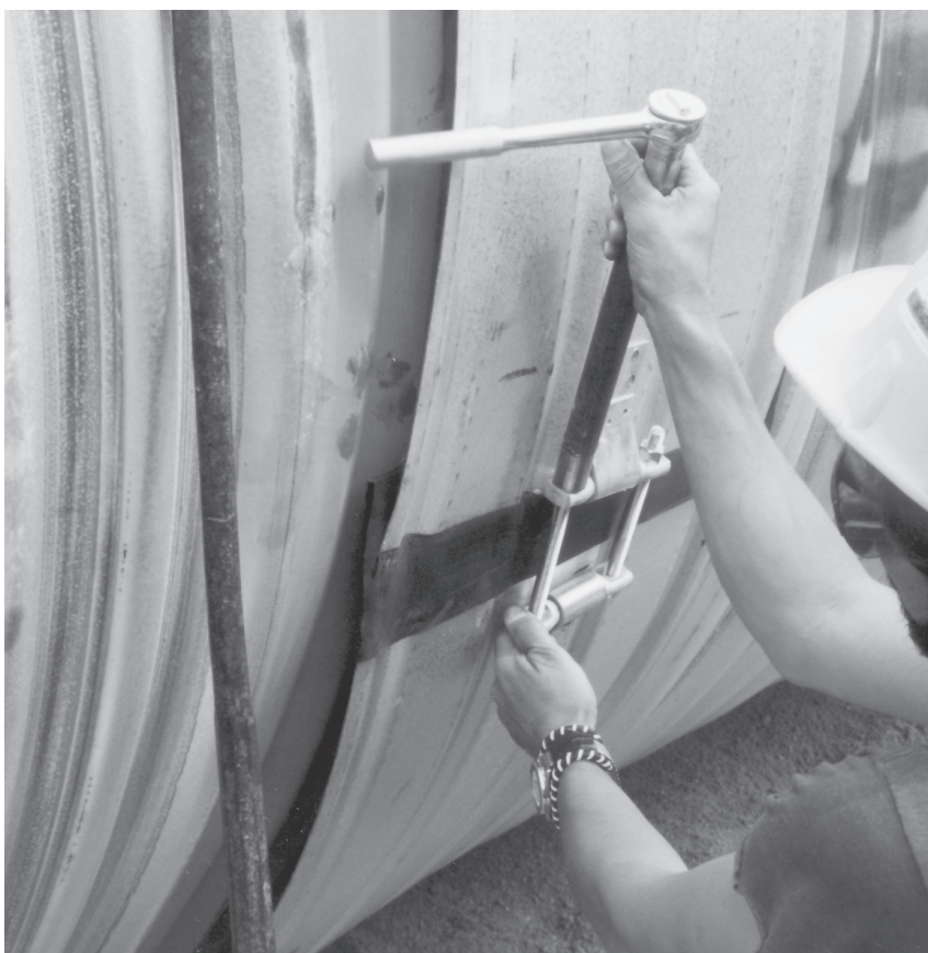
Semi-corrugated coupler installation.
