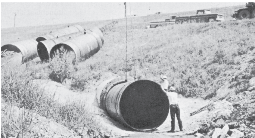
Sliplining a concrete culvert with steel pipe.
