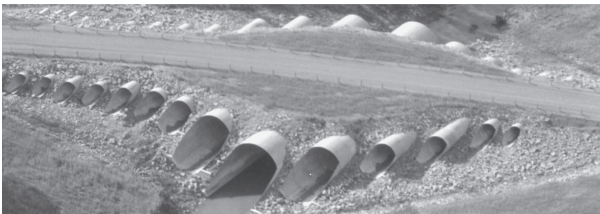
Combination stream crossing and voids to reduce dead load on foundation soils. (Ontario Ministry of Transportation project.)
