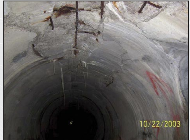
CRACKED AND CORRODED RIGID SEWER PIPE
