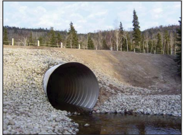
EMERGENCY REPLACEMENT FLOODED BOX CULVERT WITH CSP
