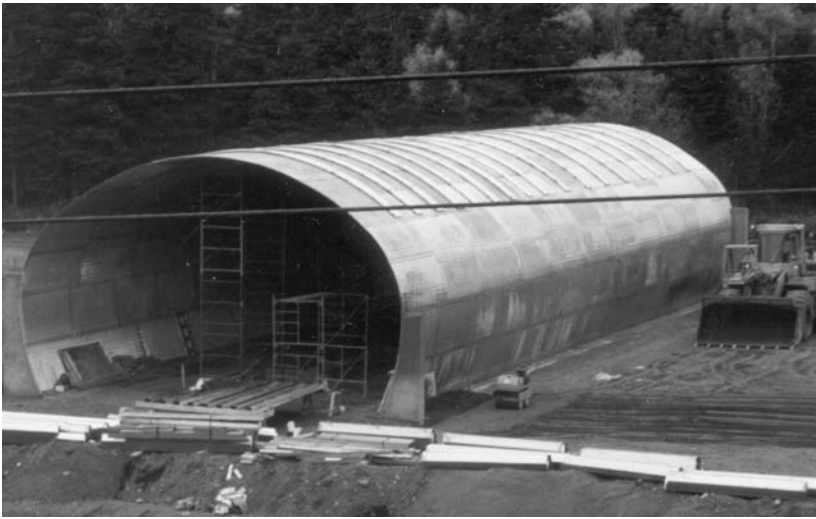
High profile arch completed assembly.
