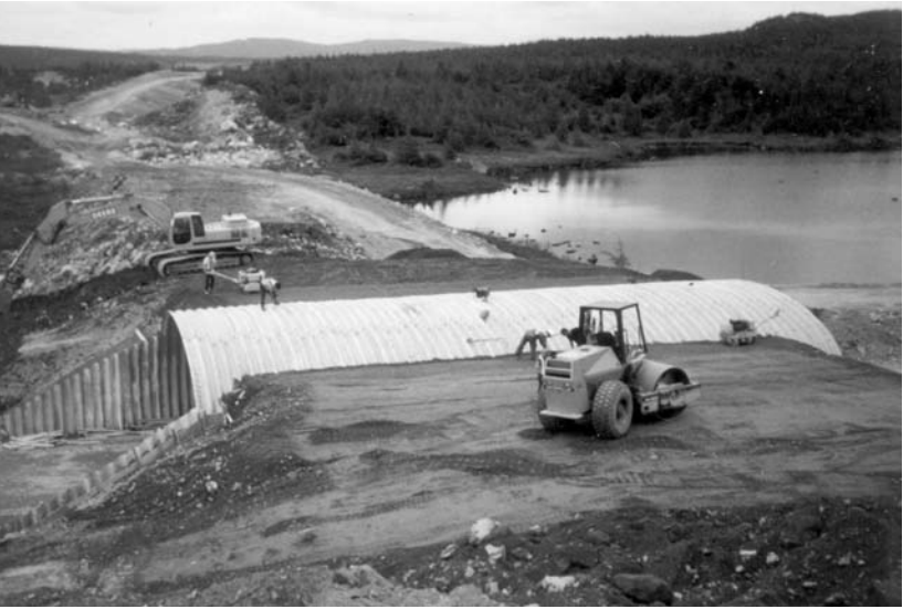
Large structure under construction.
