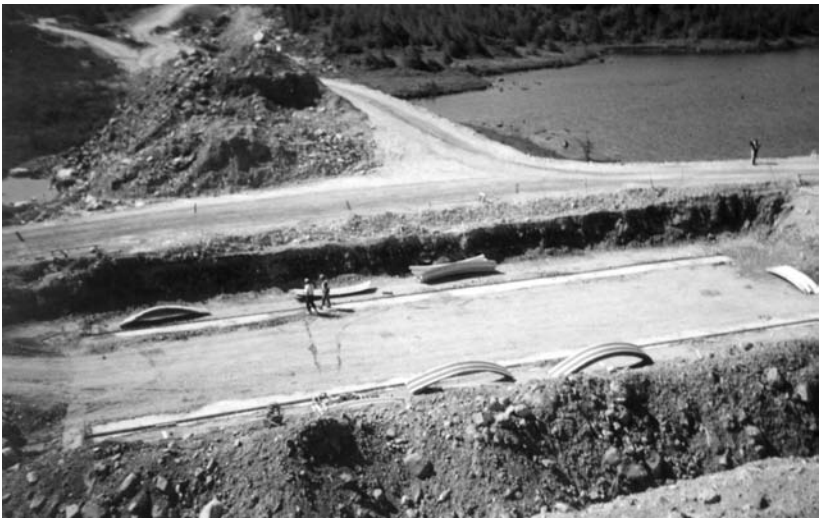
Foundation prepared for large structure.
