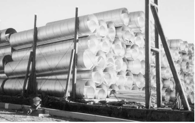
CSP for storm drainage project.
