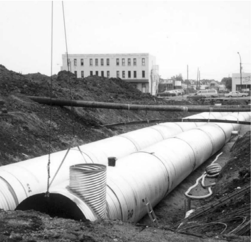
Stormwater detention tank.
