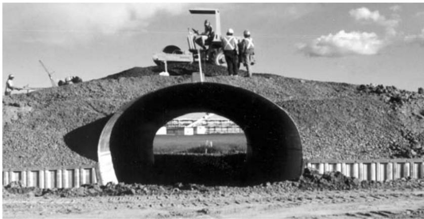
Compacting backfill over high-profile arch.
