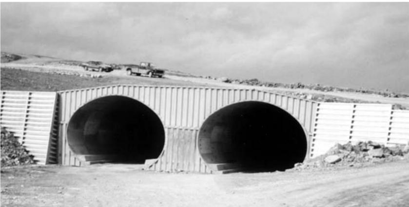
Twin high-profile arch mine underpass, with sheeting and bin-type retaining wall end treatment.
