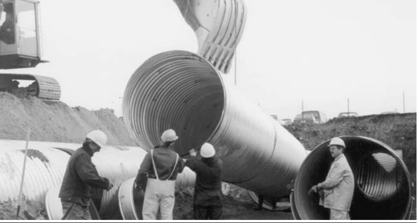
Lifting CSP into place.
