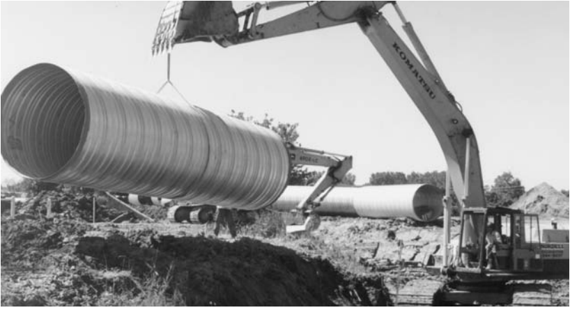
Lifting spiral rib pipe into place.
