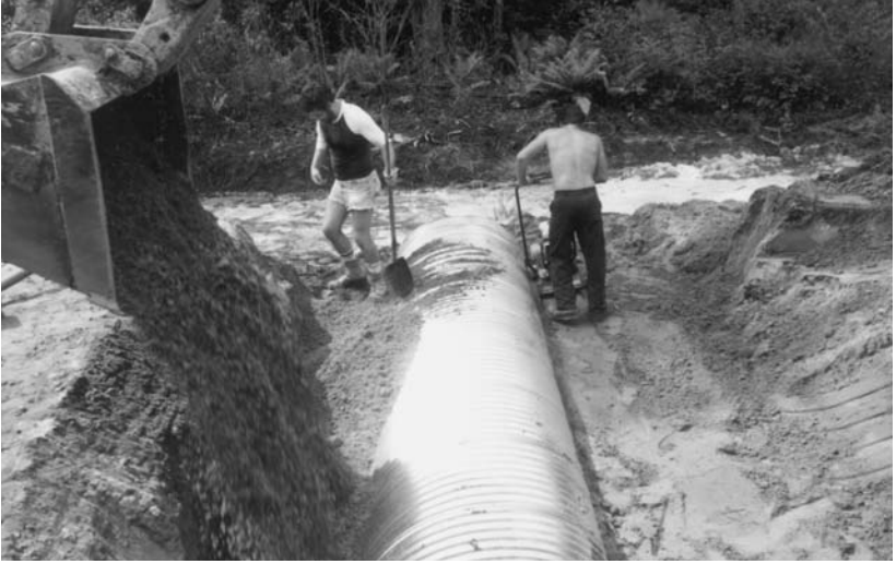
Backfill placement and compaction.
