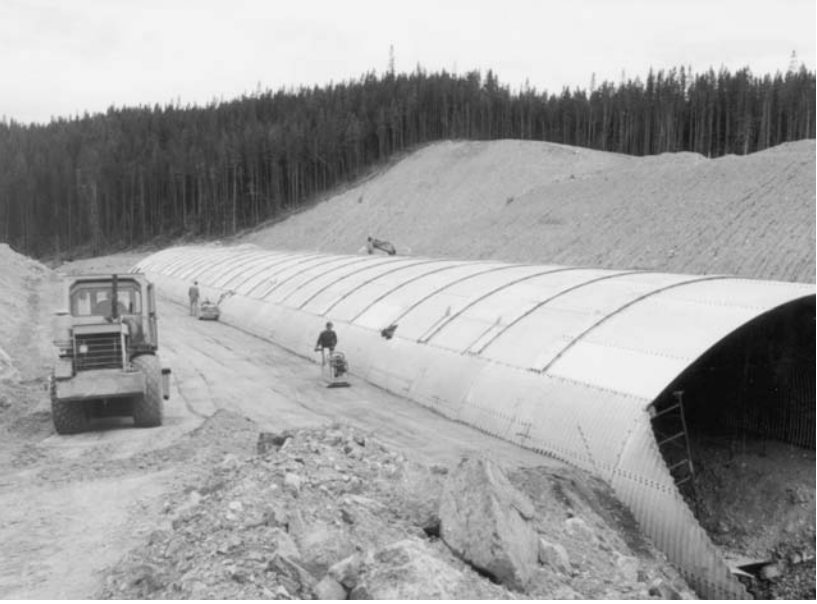
Backfill proceeds parallel to structure.
