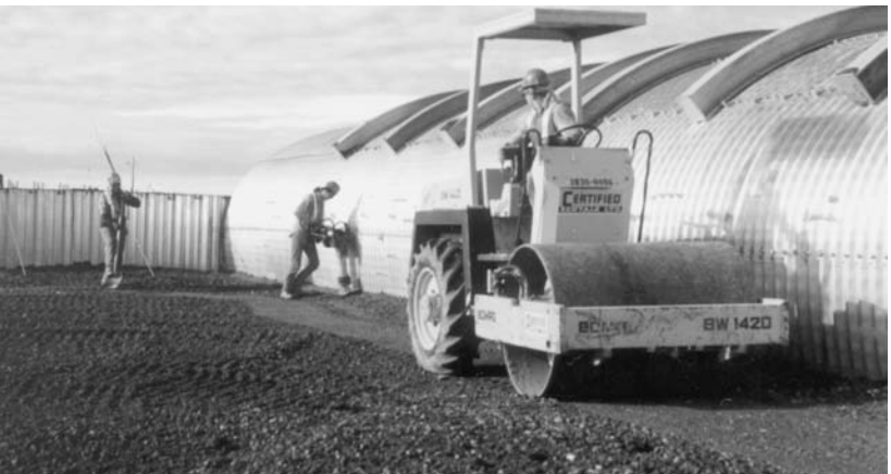
Backfill compaction adjacent to long span structural plate.
