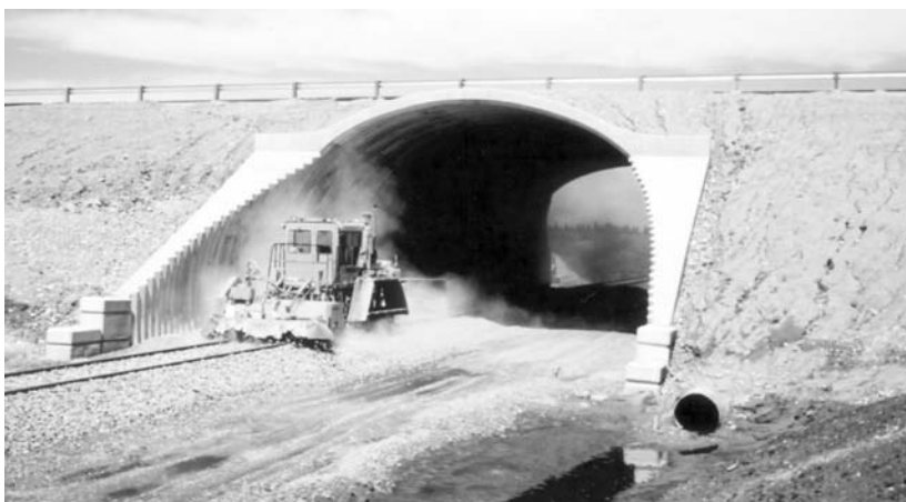
End treatment of large structure.
