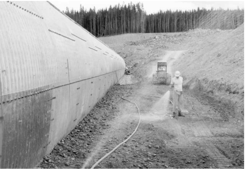
Adding water to bring backfill to optimum moisture content
