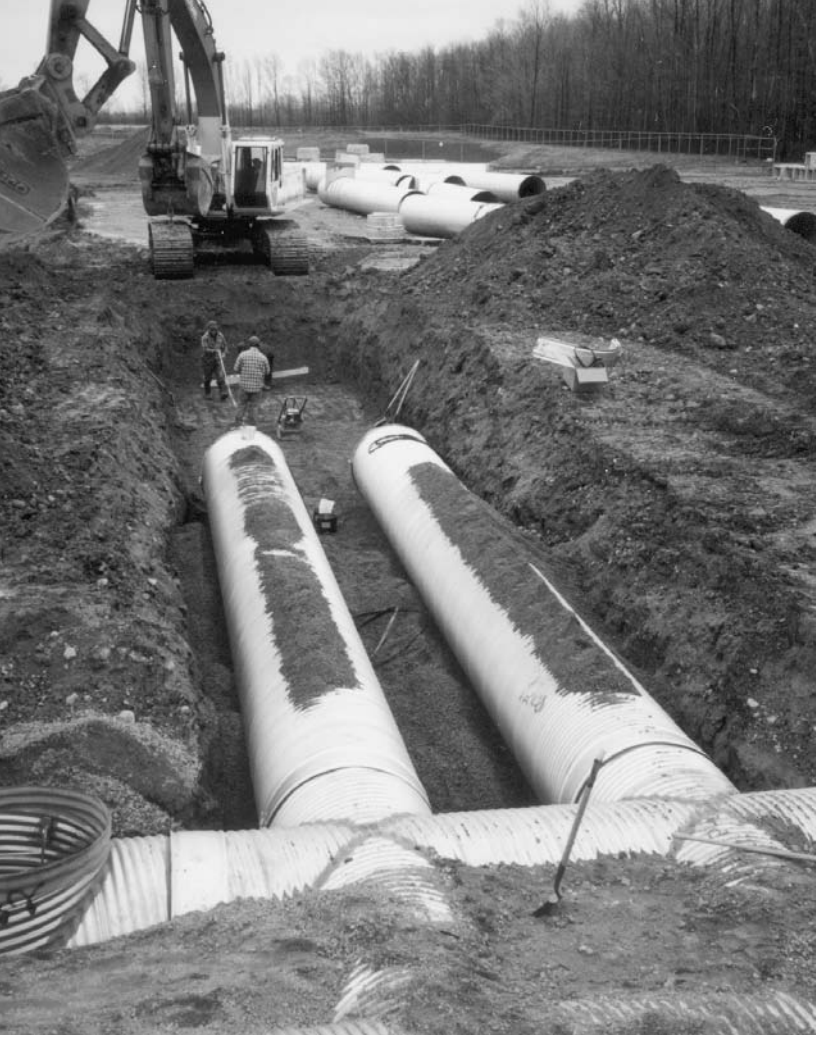
Stormwater detention system installation.
