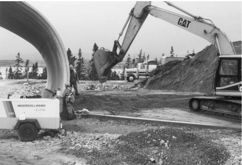
Construction of large arch.
