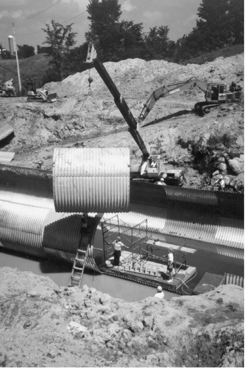
Plate assembly done from a raft.
