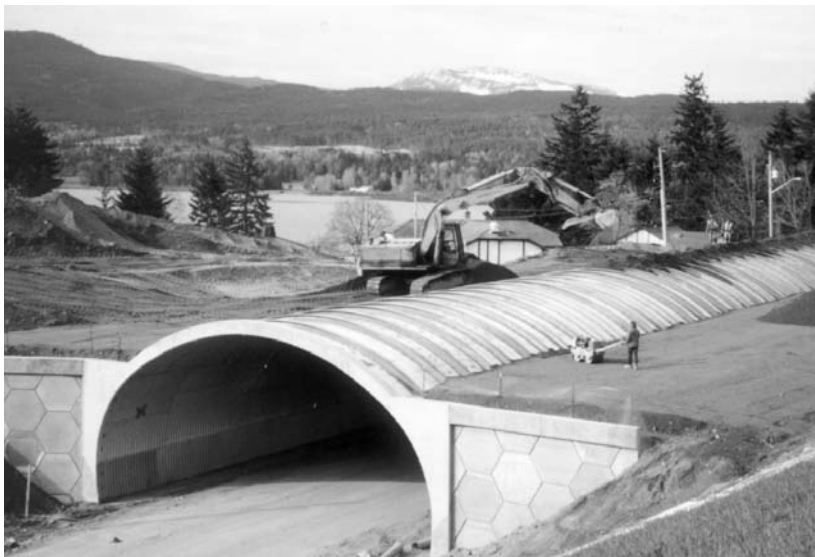
Backfilling high-profile highway underpass.
