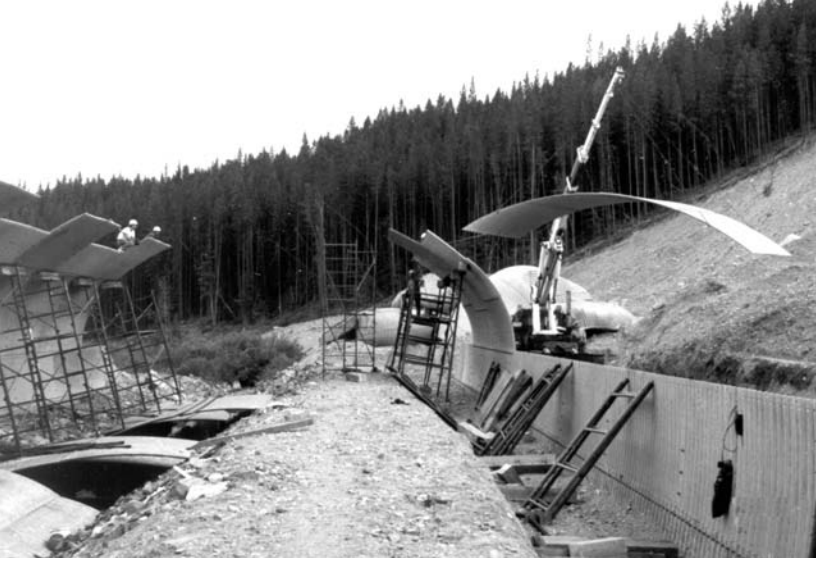
Lifting pre-assembled side plates into place.
