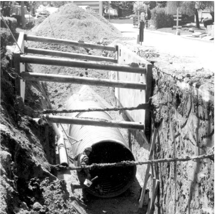
Stormwater detention tank installation in the City of Toronto.
