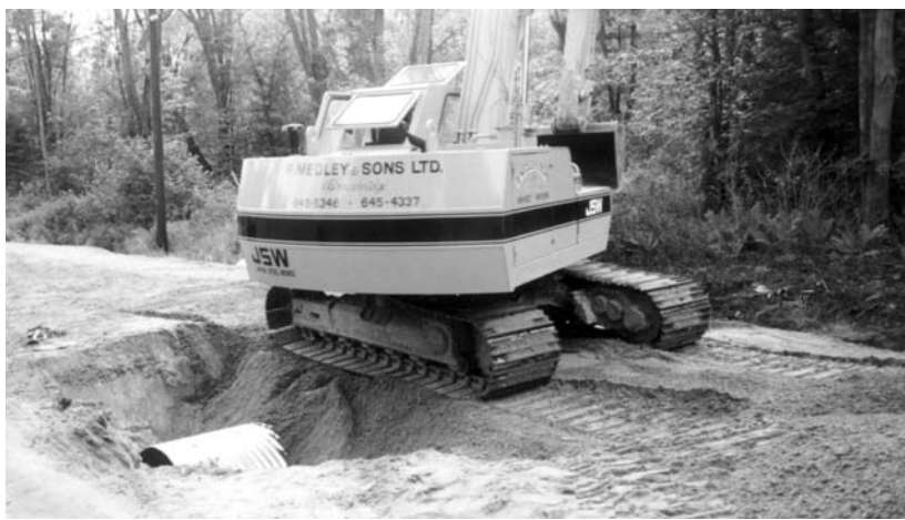
Construction load on pipe.
