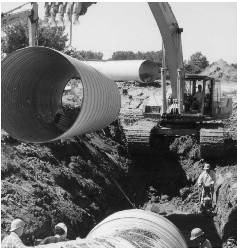
Lifting spiral rib pipe into place.
