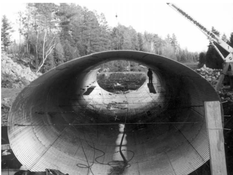
Cabing for shape control of horizontal ellipse long-span.
