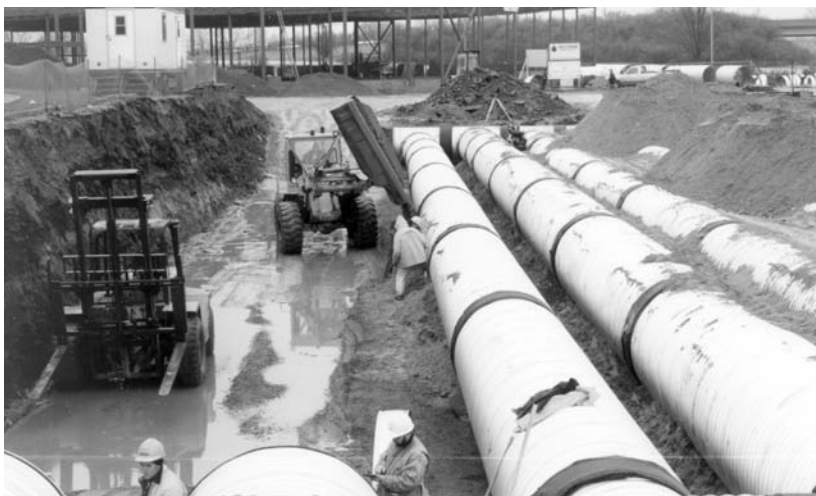
Backfilling stormwater detention system.
