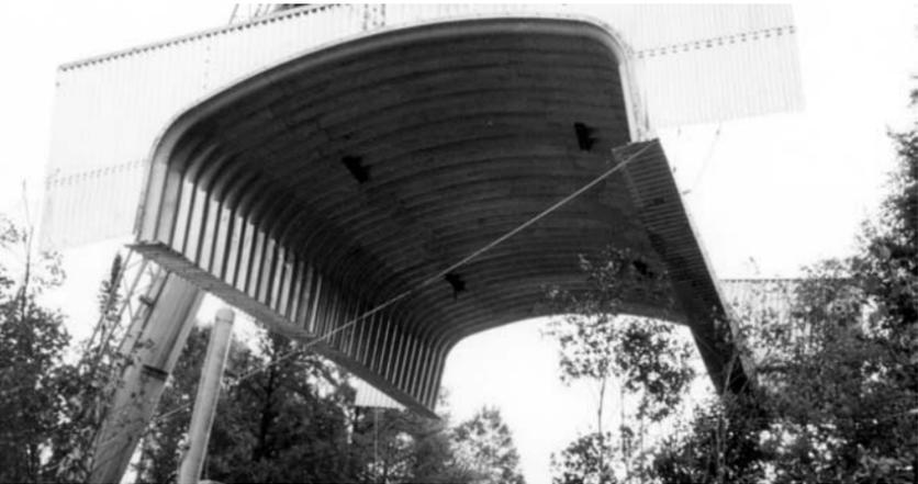
Lifting box culvert into place.
