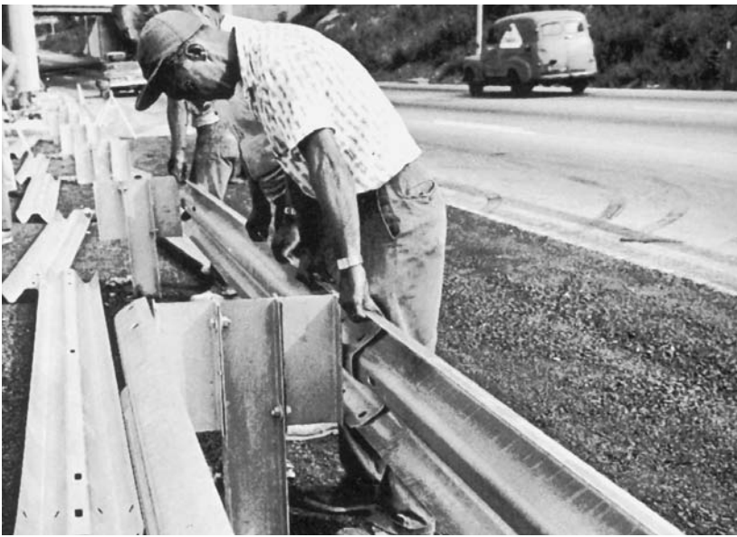
Assembly and bolting the steel guiderail joints proceeds rapidly.
