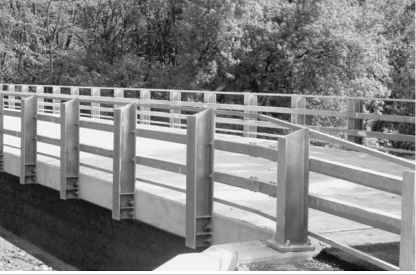
Typical bridge tubular steel railing.
