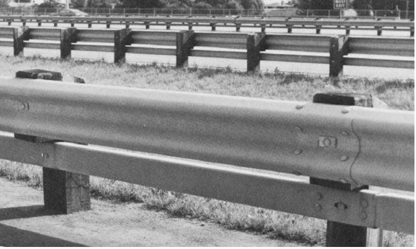
Offset mounting of W-beam on wood post.
