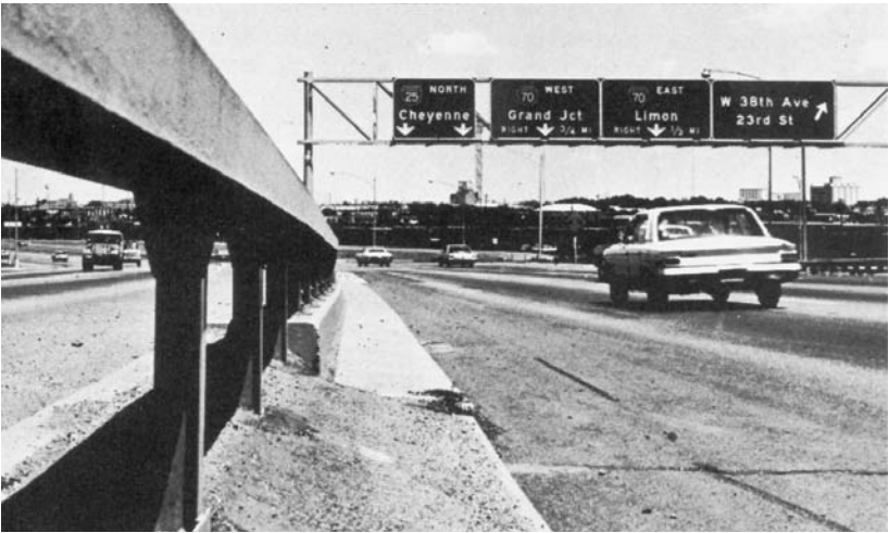
Box beam median barrier across a bridge.
