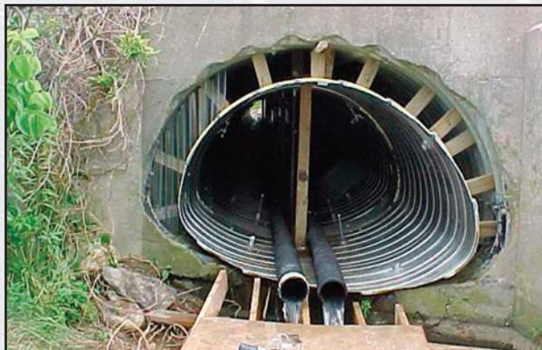
BYPASS PIPING AND END BRACING
